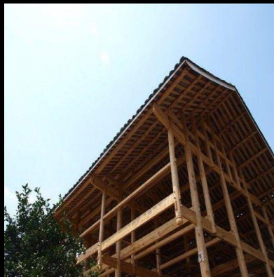
Bucket Structure 穿斗式构架
